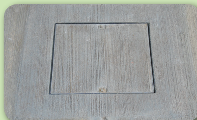
Mah Sing - 2 Storey Terrace, Rawang
